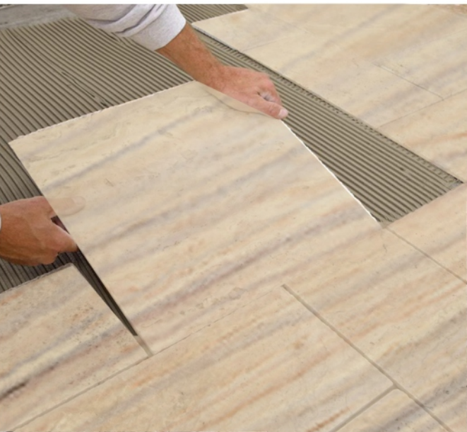
Deconyx Panels installation with silicon binding
